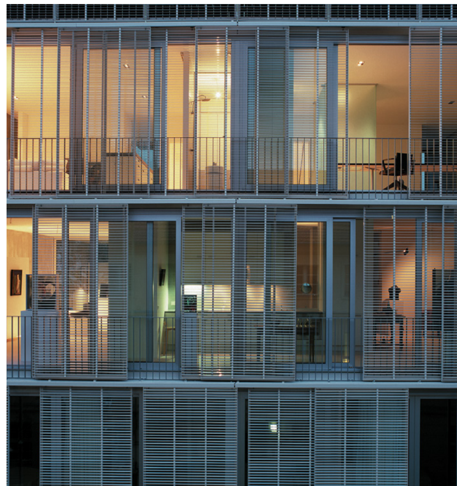
Left and above: At Urbane Living 01, Abcarius and Burns Architecture Design circumvent the prohibition of balconies by creating an operable facade. The layered facade mediates between the street and living spaces. Images: Andrea Kroth
